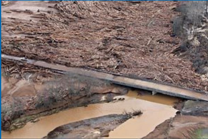
Boistfort Valley Bridge (Seattle Times)
