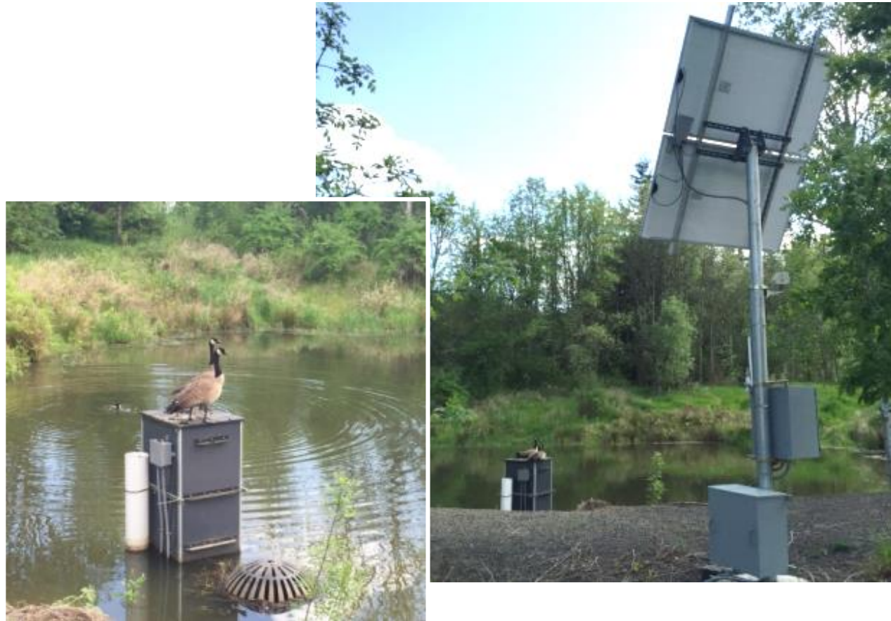
Retrofit of existing water quality facility
