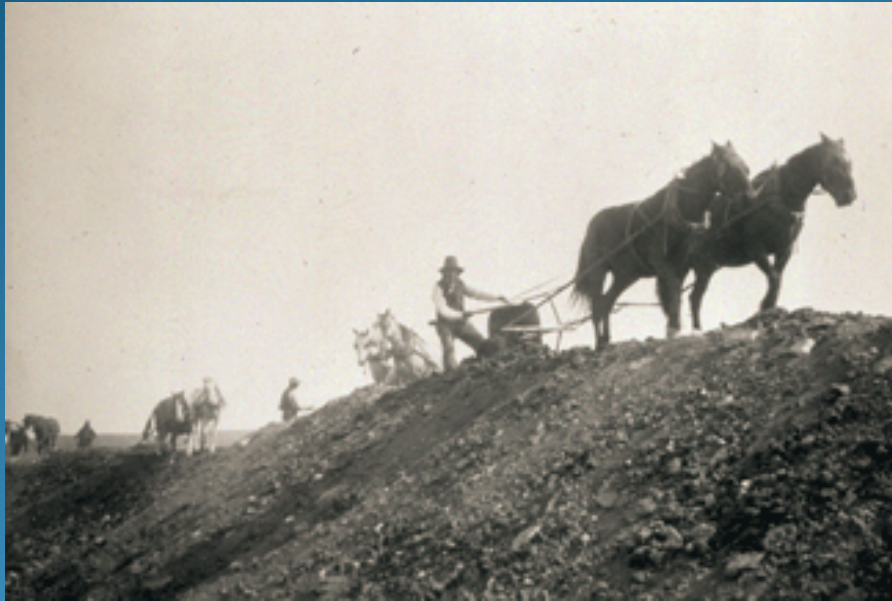
Digging the St. Mary Canal in Montana, 1908
