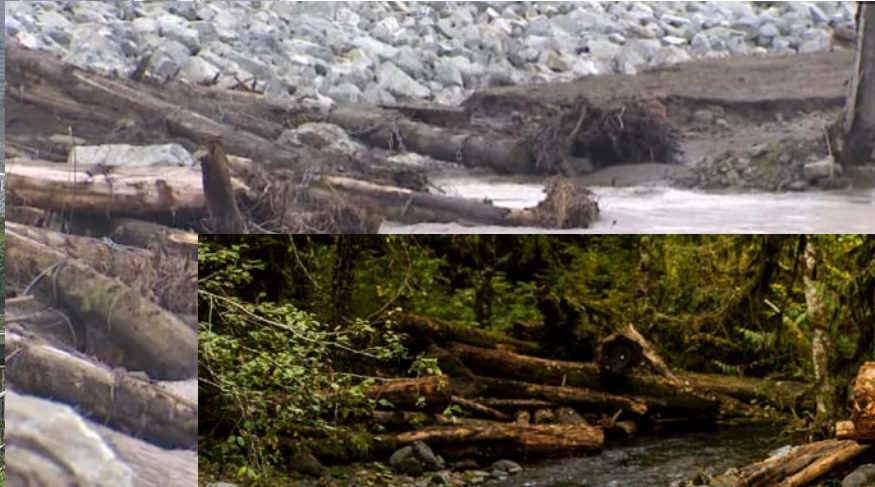
Engineered log jam, Still Creek, OR
