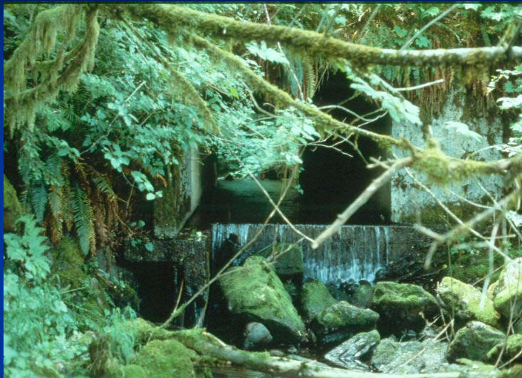
Gold Basin Site, SF Stillaguamish highway culvert pre-construction
