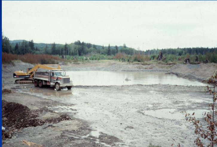
Dismal Pond, under construction
