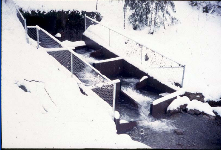
Gold Basin Site, highway culvert fishway
